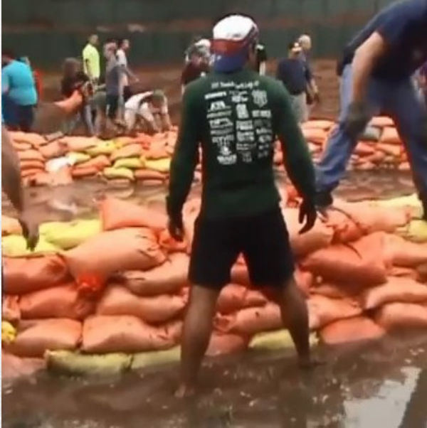
Flooding Sandbagging Along Cedar River by Waterloo Cedar Falls Courier (2016)
